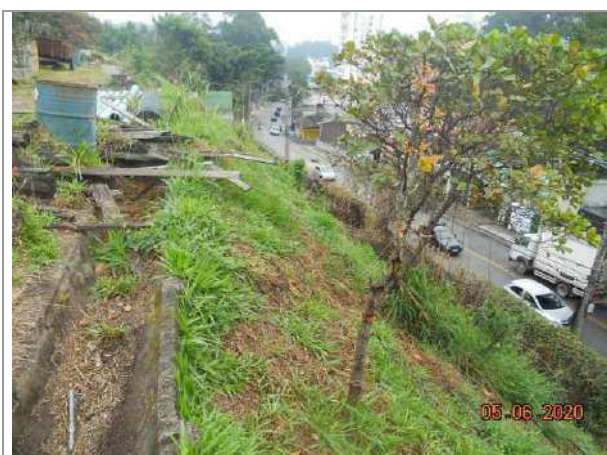
Talude recuo frontal
